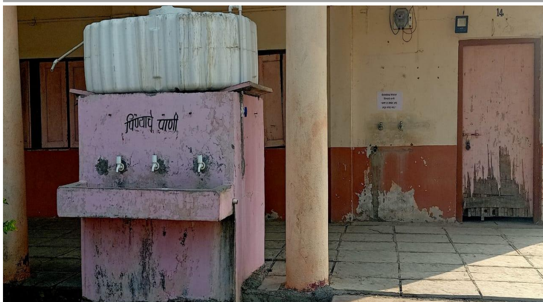
Drinking water facility
